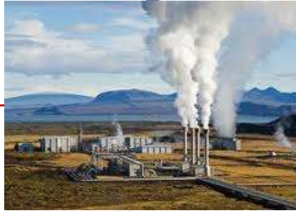
Power generation Focus area
